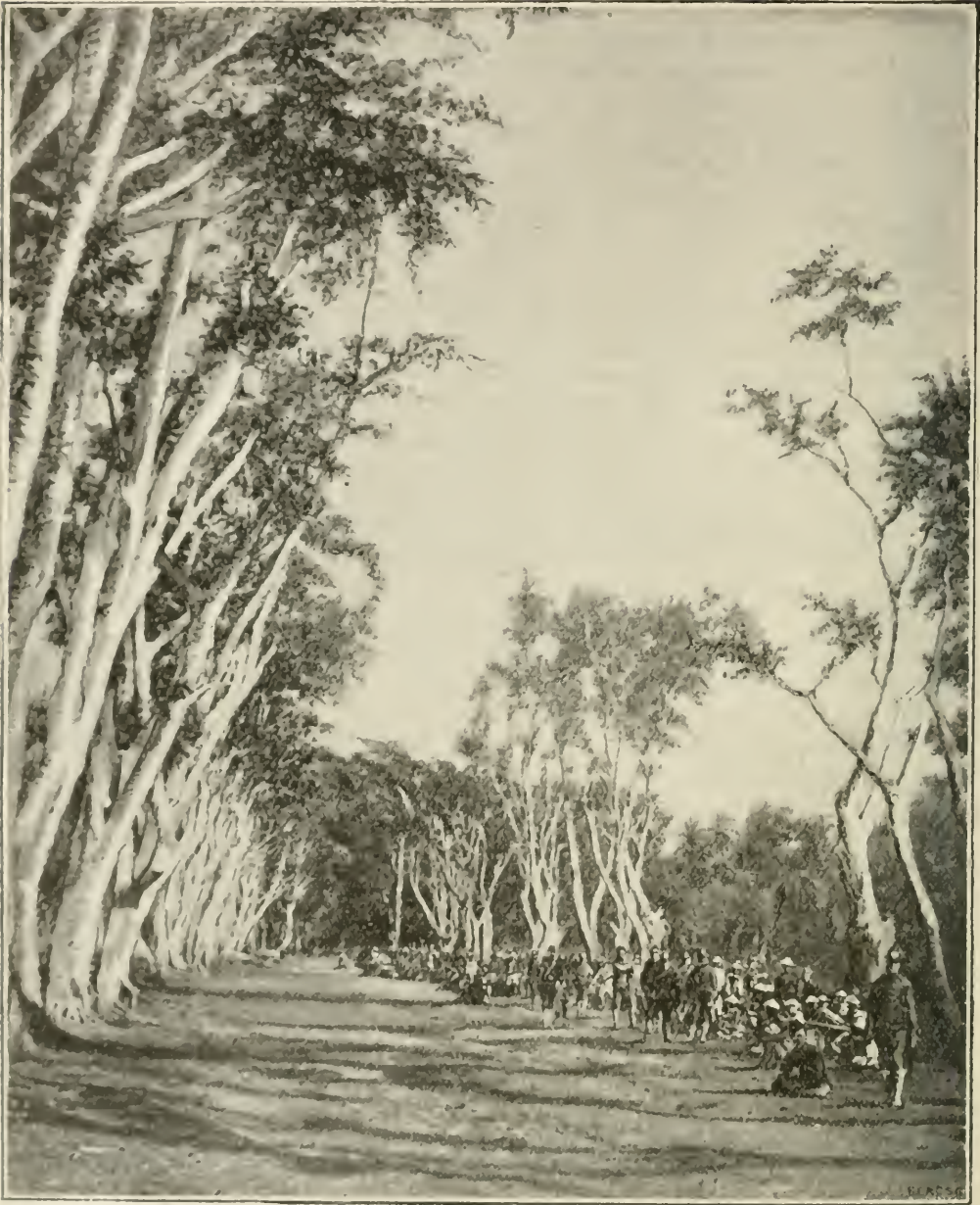
High Road from Ampanan to Mataram on 11th July.
