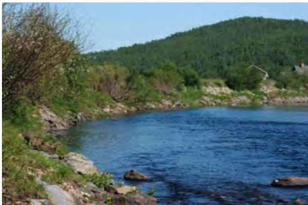
Figure 9.2 Iskuras. Before environmental measures almost completely sterile erosion control construction. Successfully re-established vegetation by transplanting vegetation mats and trees. Photo: Gunnar Kristiansen, NVE
