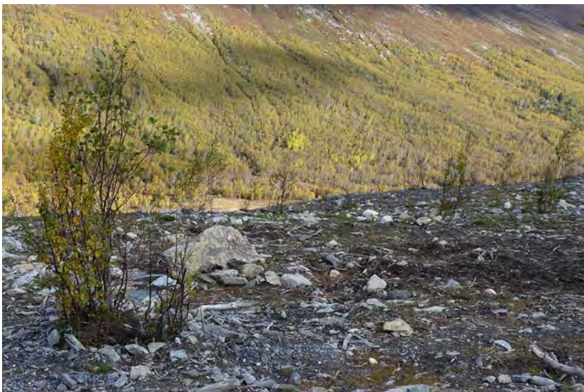
Figure 10.2 Example of transplanted turfs of vegetation and birch trees on a spoil heap covered with moraine in alpine areas in south in Norway. Photo: Arne Hamarsland, NVE
