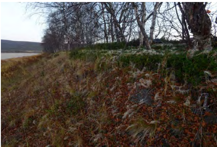
Figure12.1 Prepared slope at Hoassinjarga before installing the coir nets. The growth substrate consists of a mix of soil, organic material, silt and rocks. After a period of time vegetation is starting to establish. After 15 years the coir nets is partly and completely decomposed. The slope is stabilized and complete cover of vegetation has been established. Erosion of the slope has fully ceased. Photo: Gunnar Kristiansen, NVE
