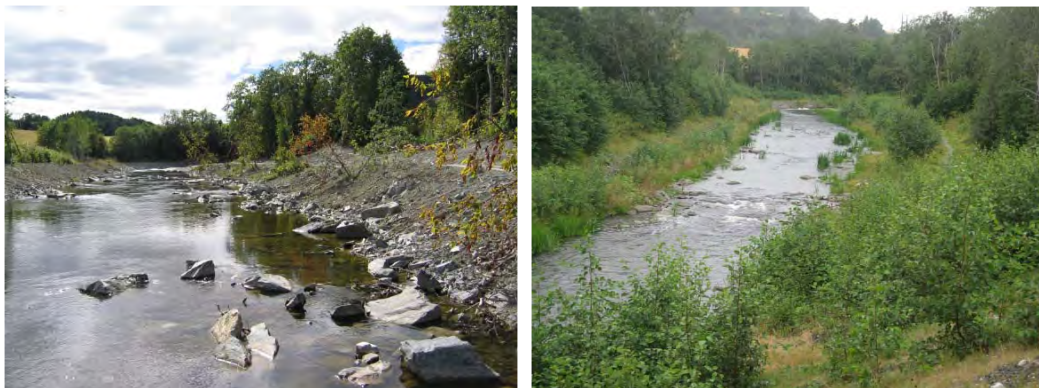
Figure 10.3 Environmental measures conducted in Vigda, Skaun involving among other methods, tree planting and transplantation. The picture to the right shows the result of the measures after only one growth season. Photo: Mads Johnsen, NVE
