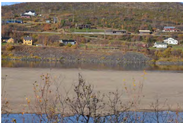
Figure 3.1.3 Example of erosion control constructions with no vegetation cover. The stone material used in the erosion control construction below is an example of a type of rocks not common along the Tana River. The color is not adjusted to the landscape and emphasizes the interventions. Photo: Gunnar Kristiansen, NVE
