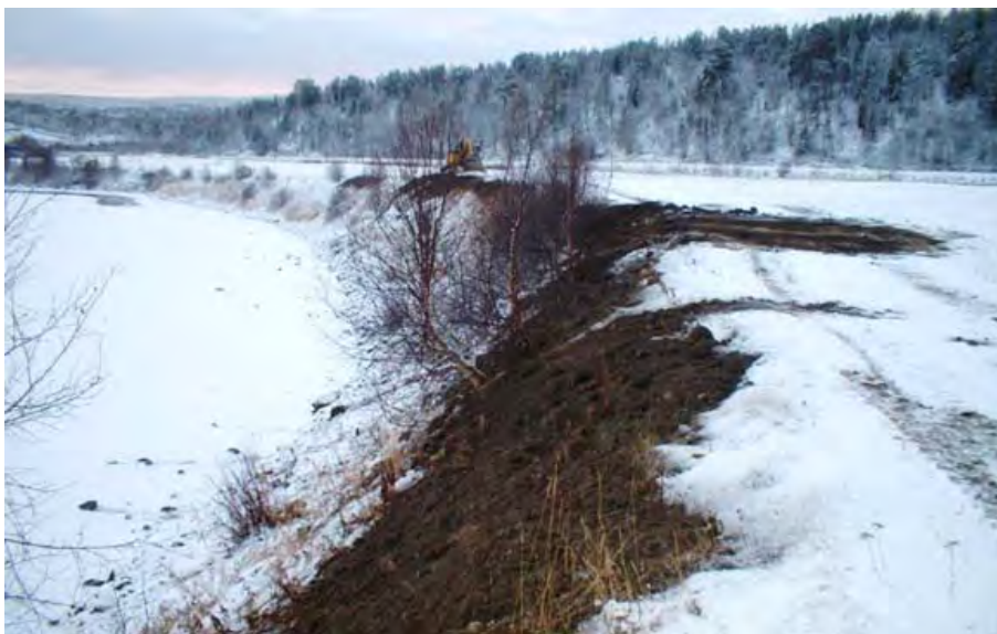
Figure 7.1 Erosion control constructions with coarse rocks, resulting in sterile and harsh environmental conditions (above). Excavator moving soil over the slope, covering the rocks with growth masses and improves the conditions for plant growth (below). Photo: Gunnar Kristiansen, NVE
