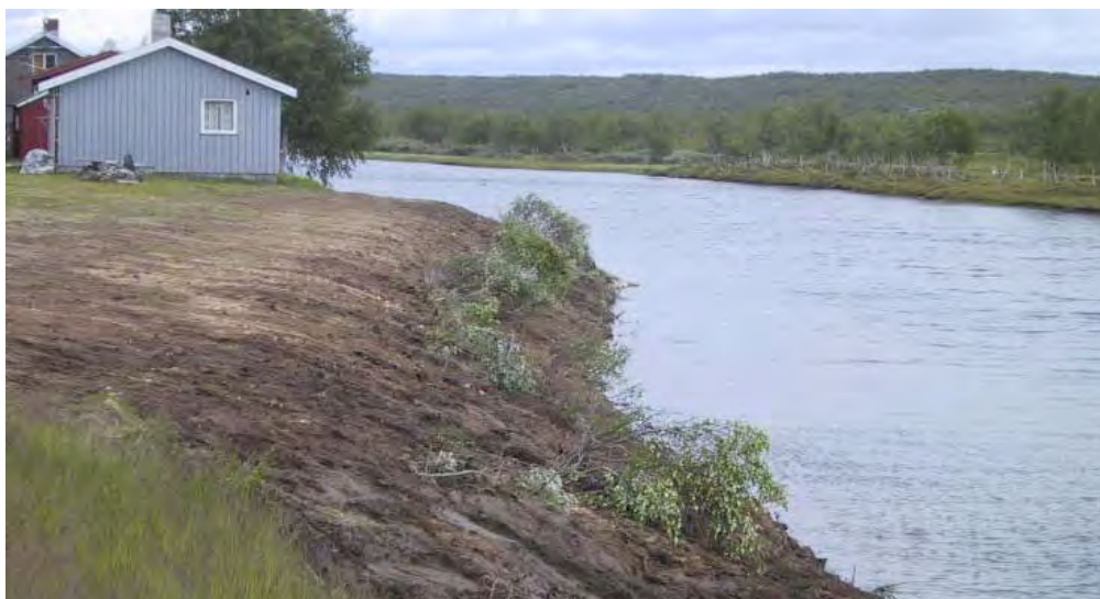
Figure 10.1 Clusters of trees and bushes moved and planted on erosion control construction at Mollisjok along Karasjohka. Photo: Gunnar Pedersen, NVE
