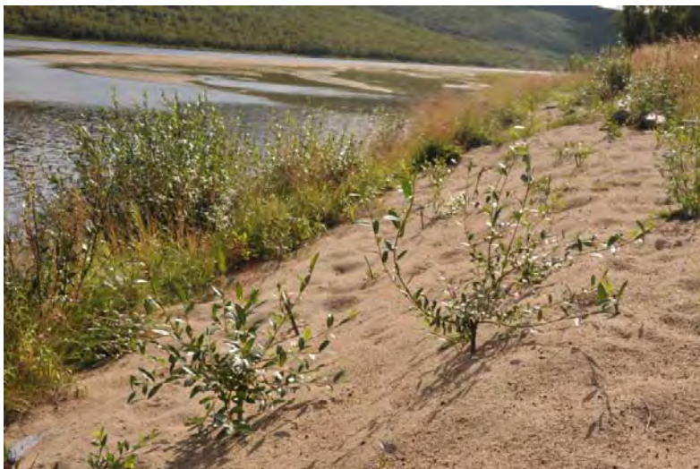
Figure 11.1 Planting cuttings directly after preparation. The cuttings are being propagated naturally in the ground and new branches are sprouting resulting in small bushes of willow, and in time forms a bush layer on the riverbank. Photo: Gunnar Kristiansen, NVE
