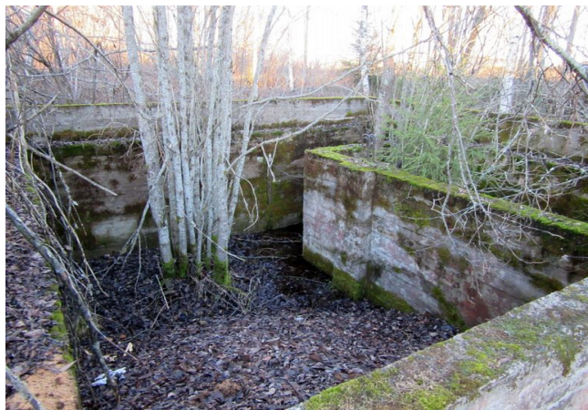
Kohde no. 2, betoniperustus.
