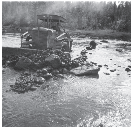
F. Stream-clearing operation with a bulldozer (1950s).
