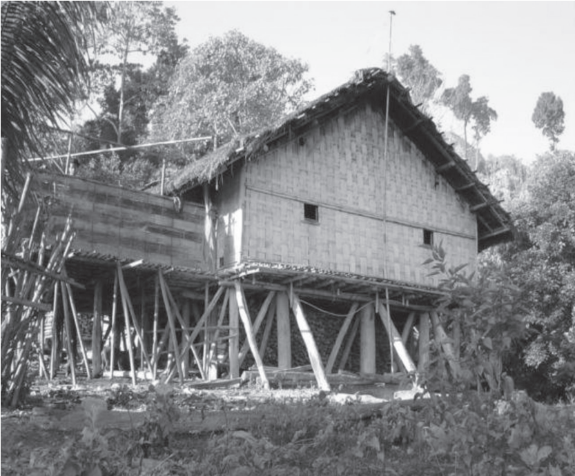
Figure 2. A Mru stilt dwelling, showing the gable end of the kim-tom and the char. Bandarban, 2003. (Photograph: Author)
