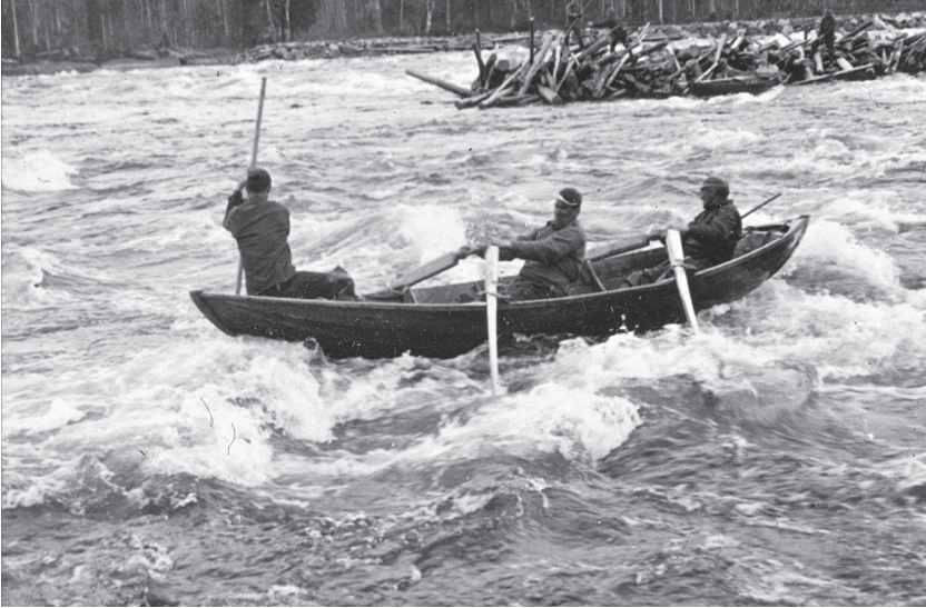
Figure 2. Practices of timber floating. Timber floaters rowing their boats in the stream. In the background, the removal of a logjam. Vindeln River, 1947.
