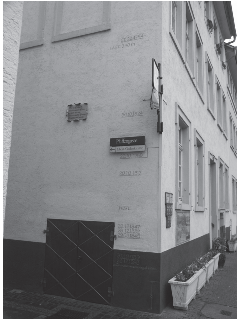
Figure 6. Flood marks in the city of Heidelberg. The flood of 1824 was the second highest of all recorded events.
