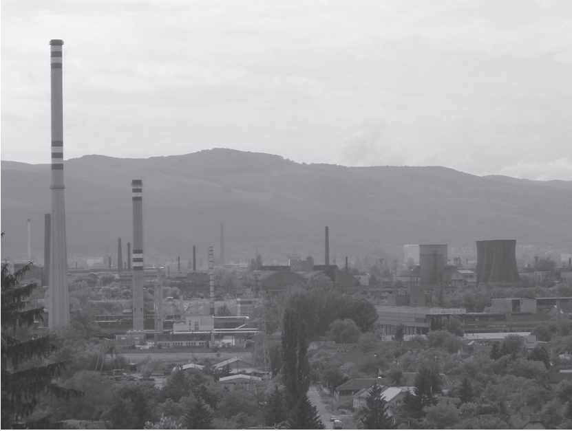
Figure 4. Closed down steelworks in Miskolc. (Photograph: Viktor Pál)
